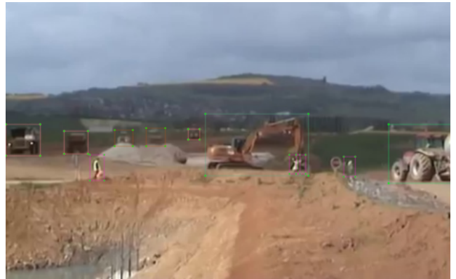
FIGURE 7. Rectangular correctly encompass ground truths: a dumper, an excavator as well as two persons. However, other trucks can be inferred from context stream frames but are not identifiable in the single image. The label should be ignored if we use YOLO v3 to detect mobile machines.
