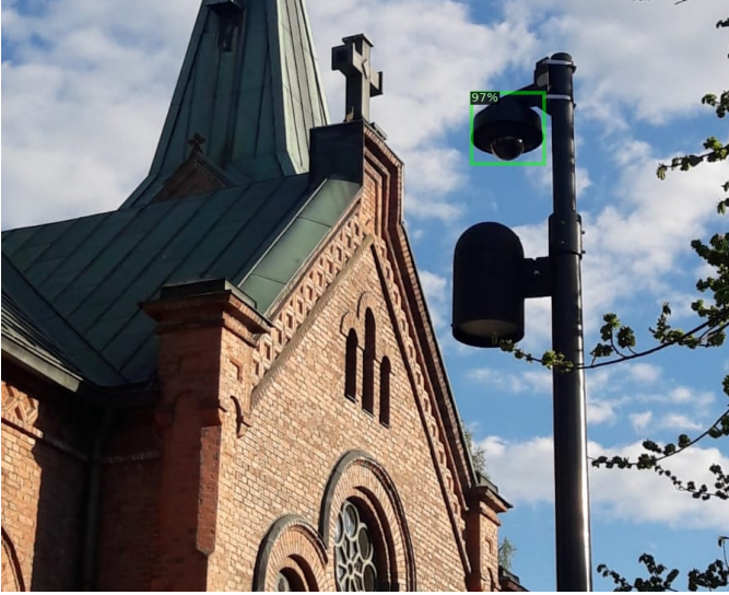
Fig. 7. Example of a hybrid installation consisting of a light pole combined with a CCTV camera. Our TridentNet model works well with a detection confidence of 97% of the “round class” instance, and avoids the potential “directed class” false positive represented by the light fixture below the camera.
