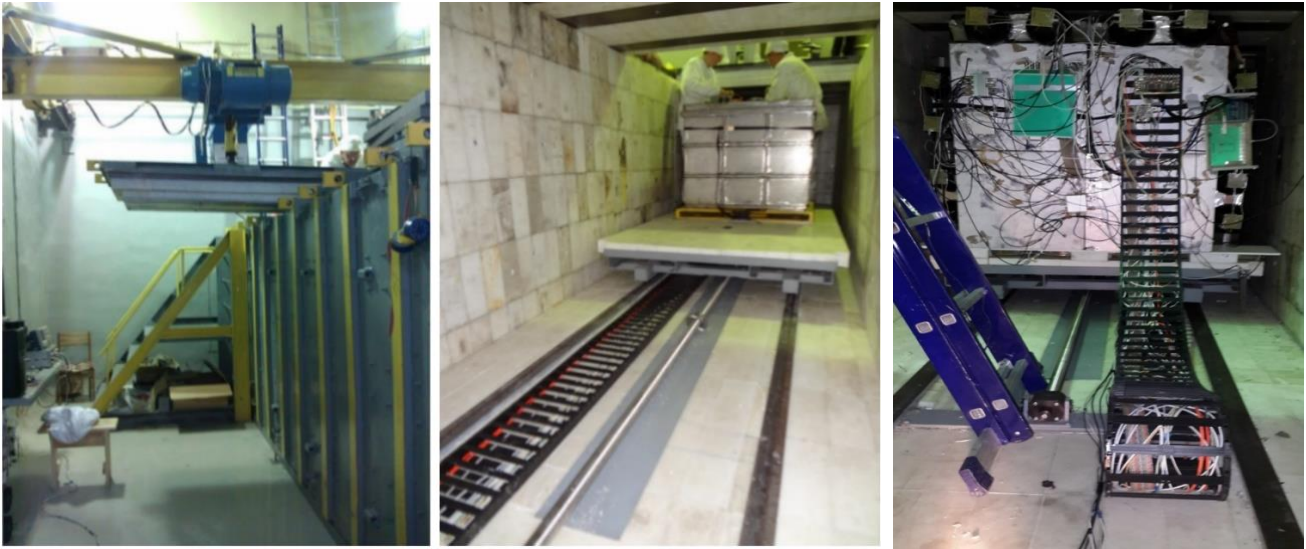
FIG. 3 General view of passive shielding: from the outside and inside. The range of detector movements is 6 - 12 m from the center of the reactor core on the left. Model detector is in the center, full-scale detector is on the right.
