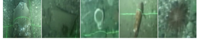
(c) Pipeline Features include an anode, grout bag, shell, fish and sea urchin.
