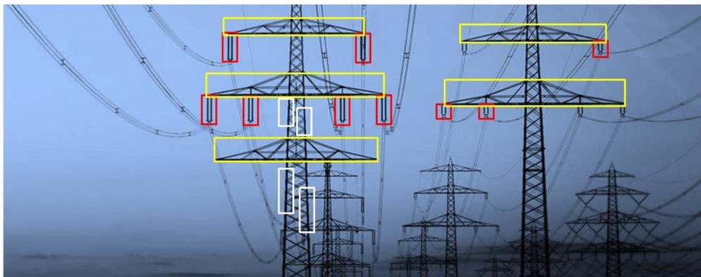
**Figure 17:** the detected insulators are surrounded by red rectangles while the structural triangles of transfer towers are surrounded by yellow rectangles. The white rectangles show the false detected features.
