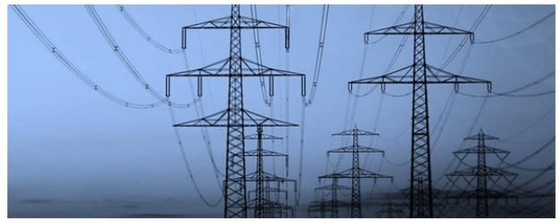
Figure 3: the conductors near to the transfer towers take the arc shape
