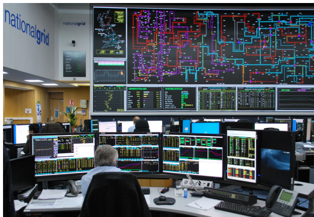
Figure 1: User-interfaces for power grid operators facilitate situation awareness, by providing information from which the power grid operator can estimate the state and predict its evolution. The sheer volume of information warrants the use of constructive tools (as opposed to ad-hoc guidelines) to synthesize the information content of the interface. Image licensed under CC BY-ND 2.0.
