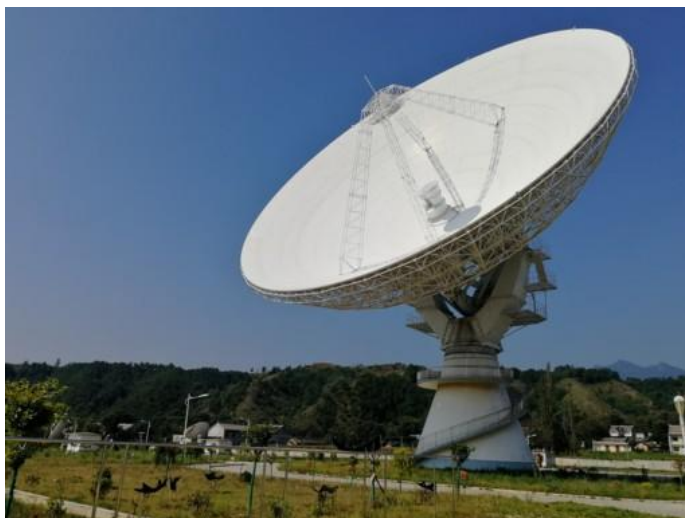
Fig. 2: The close view of Haoping 40-meter Radio Telescope.
