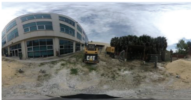
Figure 8: Cinemagraphs for site inspection (Photo courtesy Ekta Jain).
