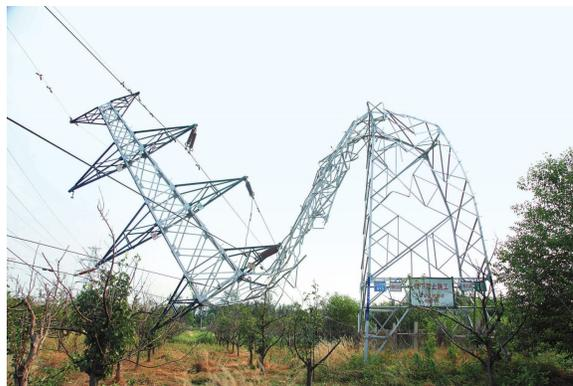
Fig. 1. Pole collapse induced by conductor galloping [4].
