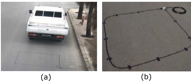
Fig. 2. (a) saw-cut loop [20]; (b) preformed loop [48].
