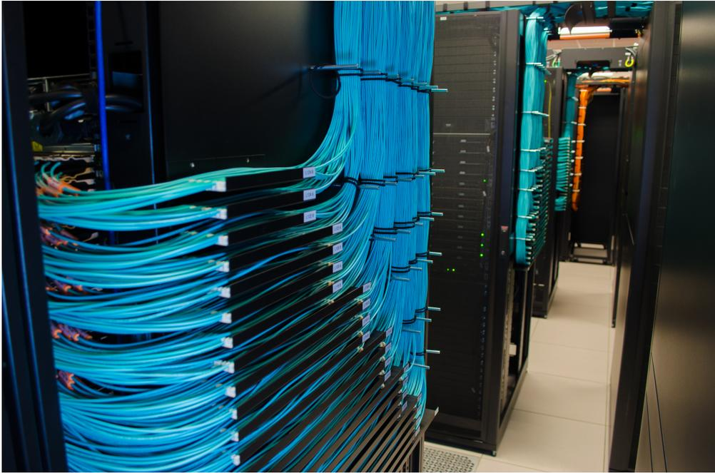
Figure 6: Networks switches for the TACC Stampede2 cluster (image courtesy Jorge Salazar, Texas Advanced Computing Center)
