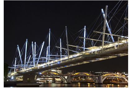
Figure 3: Kurilpa Bridge in Brisbane, Australia, is the world's largest tensegrity bridge.
