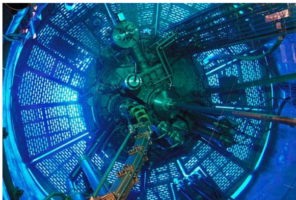
Figure 1: Top of the 58.3 MW ILL core. Blue light emanating from it is caused by the Cherenkov effect.
