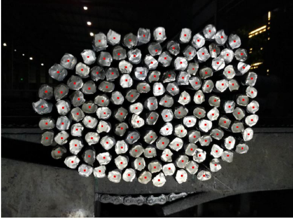
Fig. 2. An example of center localization. Red points are the centers of steel bars.
