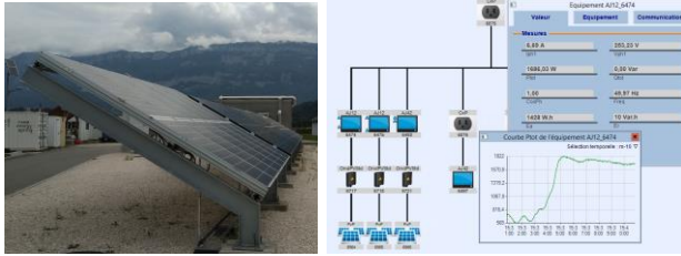
Figure 5: The smart building in consideration and its SCADA interface.
