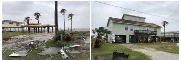
Figure 10. Post-disaster building reconnaissance images of two different houses after Hurricane Harvey.
