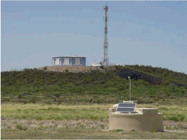
Figure 9: Photograph of a water Cherenkov detector (foreground) and a building housing six fluorescence telescopes (background) of the Auger infrastructure. Picture provided by the Auger Collaboration.
