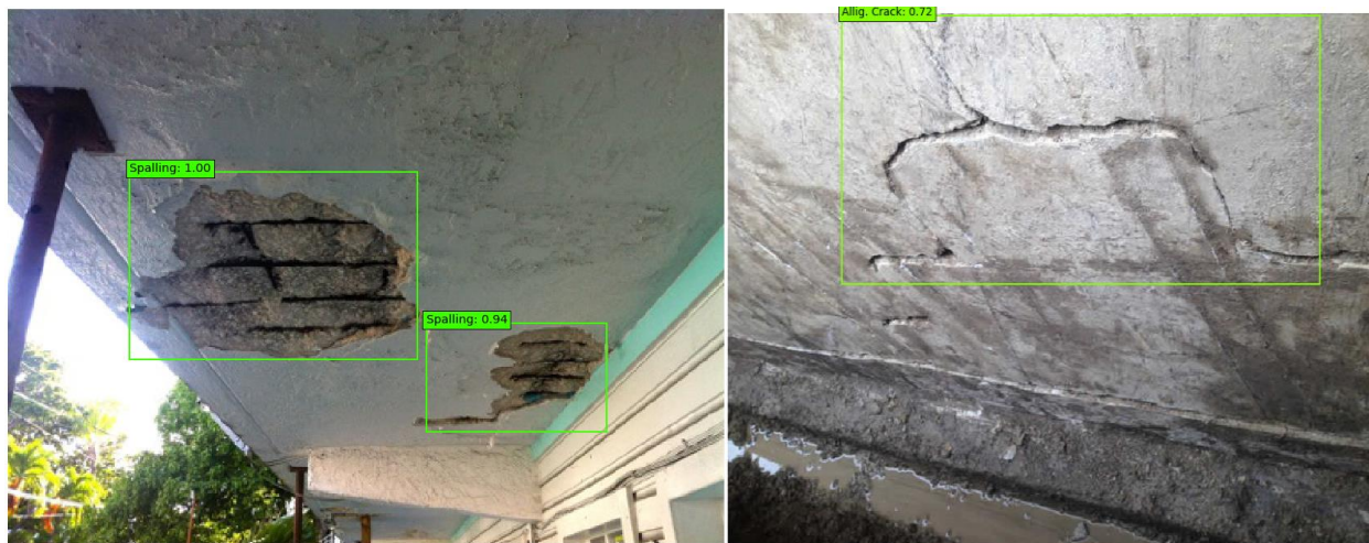
Figure 7 Damage detections on real-world images (Left: Spalling in multi locations at different depth, Right: Alligator crack detected at large angle on wetted concrete surface).
