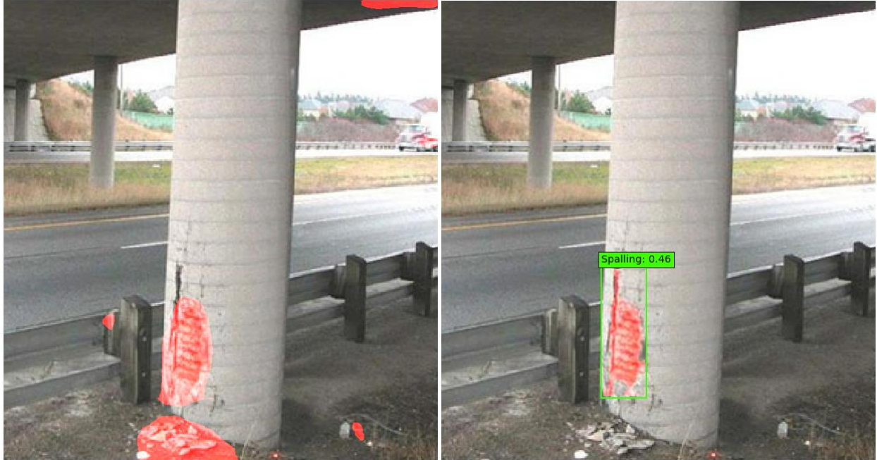
Figure 9 Effectiveness of attention guided segmentation shown in red highlighted areas (Left: Segmentation resulted in some false positive results; Right: Attention guidance readily removes misclassified pixels).
