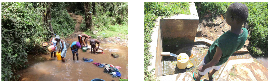
Figure 2: Images from the Busia district of Western Kenya, where 43% of individuals access water for drinking and cooking from unprotected springs (left). International Child Support, a local NGO, builds concrete structures (right) for residents to access cleaner water. From https://www.povertyactionlab.org/evaluation/cleaning-springs-kenya .
