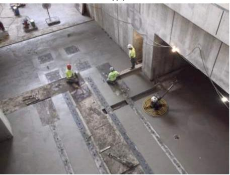
Figure 7.14. Looking down on the Mu2e detector hall. Equipment alcove A is to the right. Towards the top of the picture within the alcove, a square outline of the DT generator bunker is visible, with a trench extending out to the hall and another trench following the top wall of the alcove. There is a larger covered longitudinal trench connected where the source trench terminates near the center of the hall.
