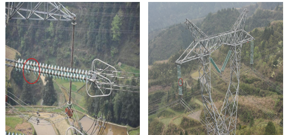
Fig. 2: The self-blast glass insulators: the broken parts are labelled by red circle.
