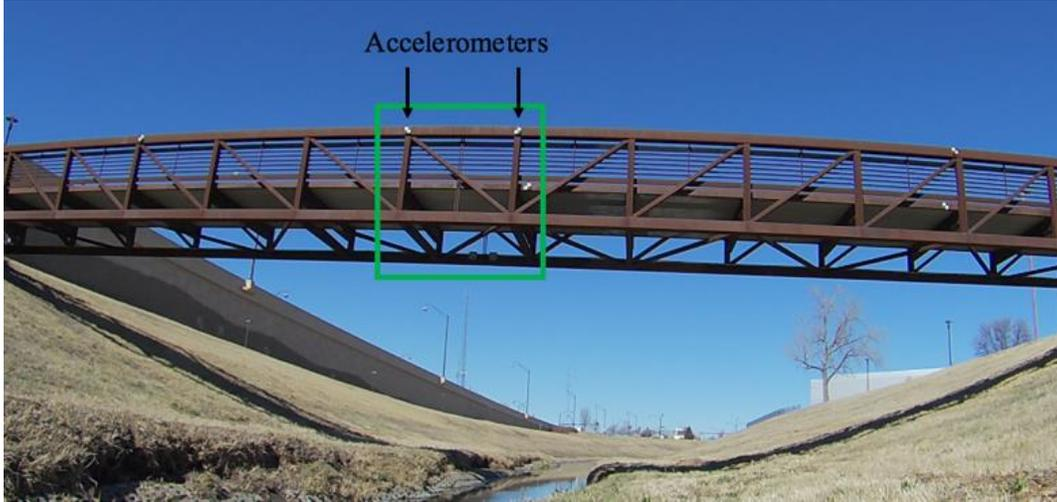
Figure 5 The pedestrian bridge, location of accelerometers and camera view (green rectangle) are marked
