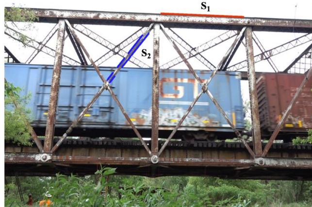
Figure 7 Image view of the railway bridge along with feature points extracted from structure S1(in red) and S2(in blue)
