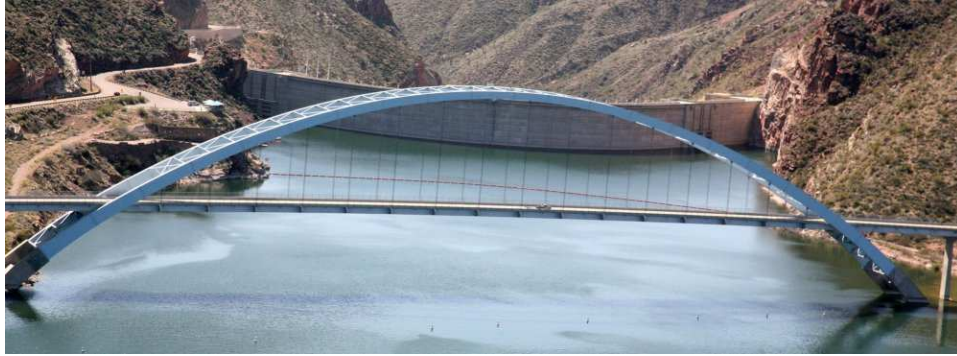
(a) Picture of the bridge with the dam accelerating winds in the background.
