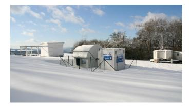
Figure 1: Projectsoft BlueEye600 robotic observatory located in Ondřejov, Czech Republic. The alt-azimuth telescope is of Ritchey–Chrétien type with the primary diameter d = 600 mm.
