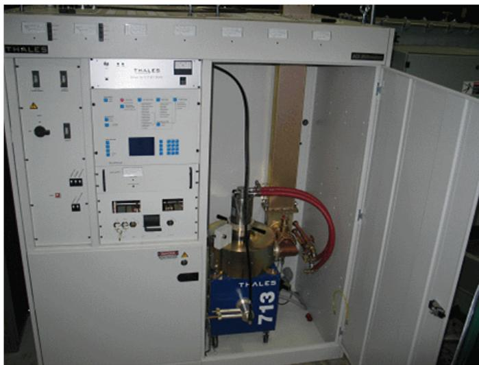
Figure 4.4.3: IOT inside the transmitter.
