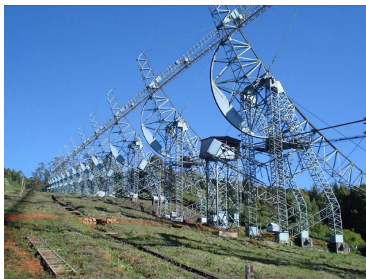
Figure 1. The Ooty Radio Telescope is an offset cylindrical paraboloid, 530mx30m in size. It is equatorially mounted. The Ooty Wide Field Array (OWFA) is an upgrade to the ORT, which digitizes the signals from every 4 dipoles along the feed line. These signals are then cross-correlated, leading to a very wide field of view interferometer. See the text for more details.
