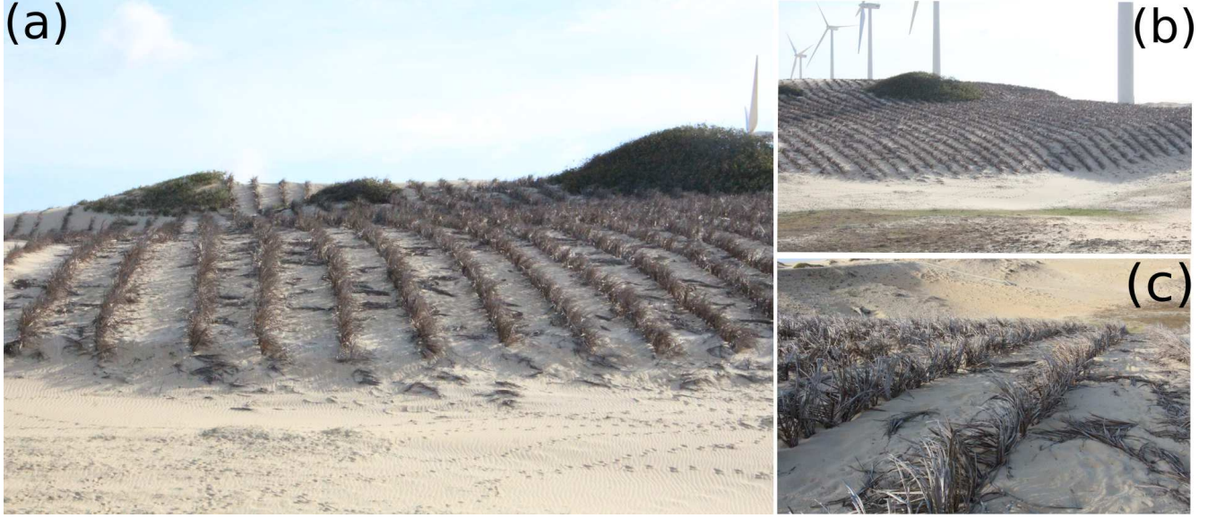
Figure 1. Application of sand fences to prevent wind erosion — a field example. The images (a)-(c) show fences made of coconut leaves in Paracuru, near Fortaleza, main city of State of Ceará in Northeastern Brazil (photo by first authors, I.A.L. and A.D.A.).
