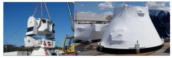
Figure 5: Left: Disassembly of the receiver cabin/yoke arms unit from the yoke traverse, before insulation work; Right: Shrink-wrap of the support cone with the azimuth bearing and lifting fixture integrated is in progress.
