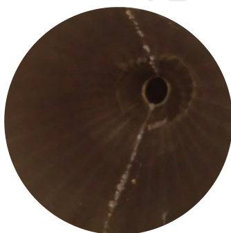
Figure 7. Internal surface of the Venturi-tube cavitation reactor, downstream the nozzle, after about 1,000 hours of operation.
