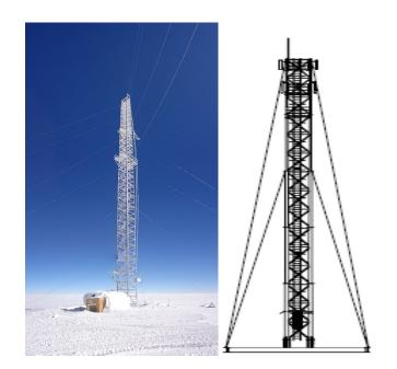
Figure 120: the "American tower" at Concordia Station, a guy-cable tower (left); a schematic of a tower with less footprint but with a basement loaded with concrete (right, courtesy of ITAS company) -iving docume
