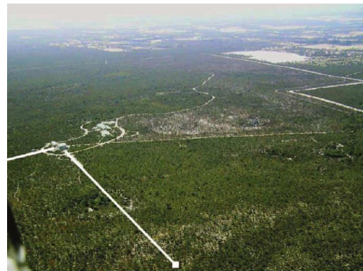
Figure 6 (Color online) Aerial photos of the flat sand plain proposed as a site for a future southern hemisphere GW detector. The proposed long arms are added in this photo.
