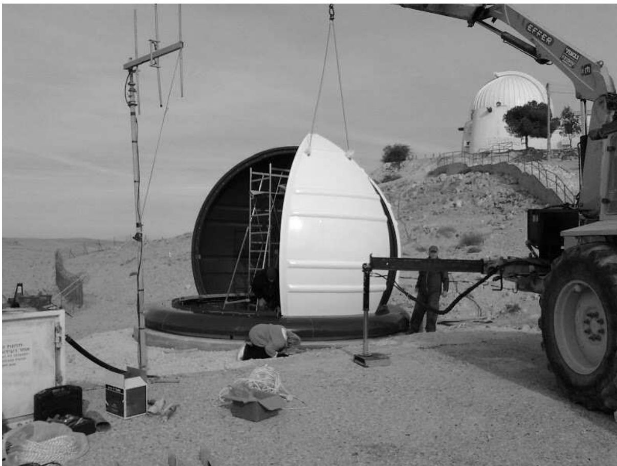
Fig. 2.— Construction of the C28IL dome. The concrete base is visible under the skirt of the partly-completed dome, while the crane is supporting one of the dome segments prior to connecting it to the rest of the dome. The antenna seen in the foreground was moved since it could, in some situations, block the telescope view.
