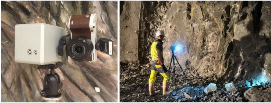
Figure 1: Left: Data acquisition system based on a consumer camera with fixed focus lens, and a stepper motor unit. Right: Typical data acquisition situation close to the hazardous region of the tunnel face.
