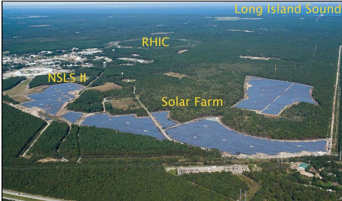
Figure 2: Aerial view of BNL with NSLS II, RHIC and the Solar Farm indicated.
