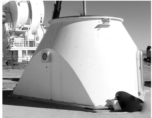
Figure 7: New support cone for the GLT showing bottom open to snow environment, full conical shape with 6 points support (left), ALMA-NA prototype antenna support cone, truncated, 3 support point (right)
