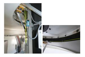
Figure 5. Photos of azimuth emergency limit switch arrangement.On the left is the pully arrangement, and on the right is the cord playout around the inside of the cable wrap room ceiling. Images courtesy of Stuart Weston
