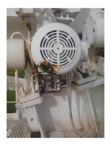
Figure 4. The state of the old motors was very poor and were considered a safety issue.
