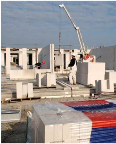
Figure 2 Building with calcium silicate elements using a dedicated crane
