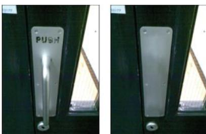
**FIGURE 1.** Poorly- and well-designed doors.<sup>8</sup>
