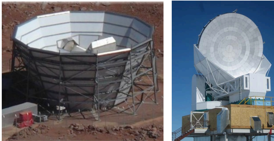
Figure 7: Left: The ACT 6 m telescope in northern Chile. The telescope is inside the 13 m tall ground screen. The secondary is just visible near the center of the ground screen. Right: The SPT 10 m telescope at the South Pole. Most of the circular primary reflector is visible, while the cryogenic secondary reflector and receiver are housed inside the white structure below and to the right of the primary. (Photos courtesy of ACT and SPT Collaborations.)
