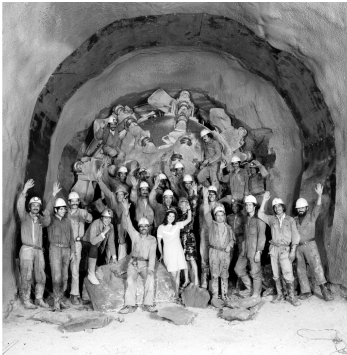
Fig. 16: The SPS ring tunnel is completed
