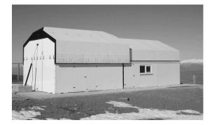
Figure 3. Reinforced glass-fiber enclosure at OAdM.
