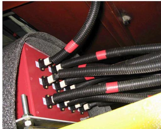
Fig. 4. Barrel distribution box. Twelve delivery fiber cables in protective tubing connect to the MTP optical fiber couplers. Each cable has 8 fibers.
