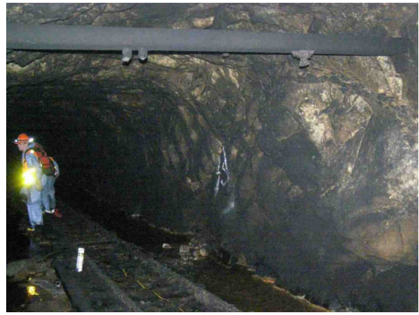
FIG. 2: Station 308 in the Pioneer Tunnel during recent reconnaissance [5].
