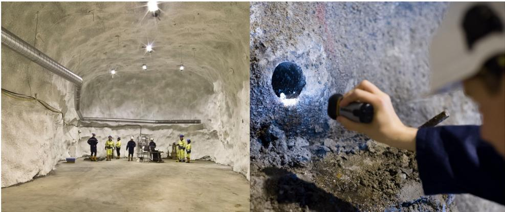
**Figure 4.** Left: the experimental hall of Callio Lab2 after its completion in the spring of 2016. The area is about 120 m<sup>2</sup>. The maximum height is 9 m. Right: example of a borehole originating from Callio Lab2. The diameter is 7.5 cm. Typical length is about 700 m. Due to the high quality of the rock, the inner surface of the hole is smooth, facilitating deployment of instrumentation. The photo was taken before the walls of the main hall were painted.
